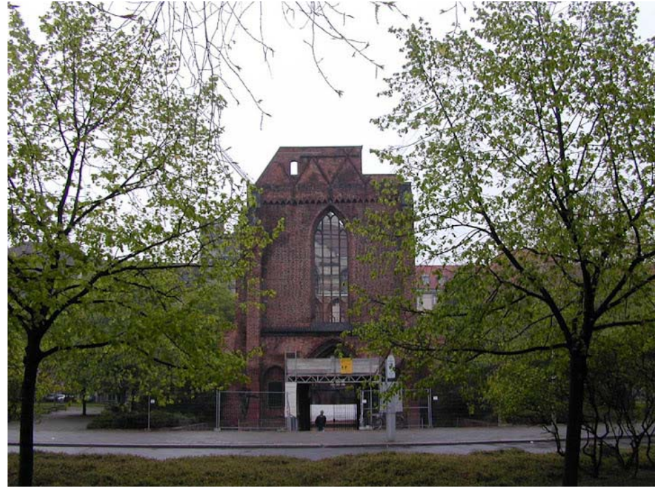
Facade of Klosterruine
