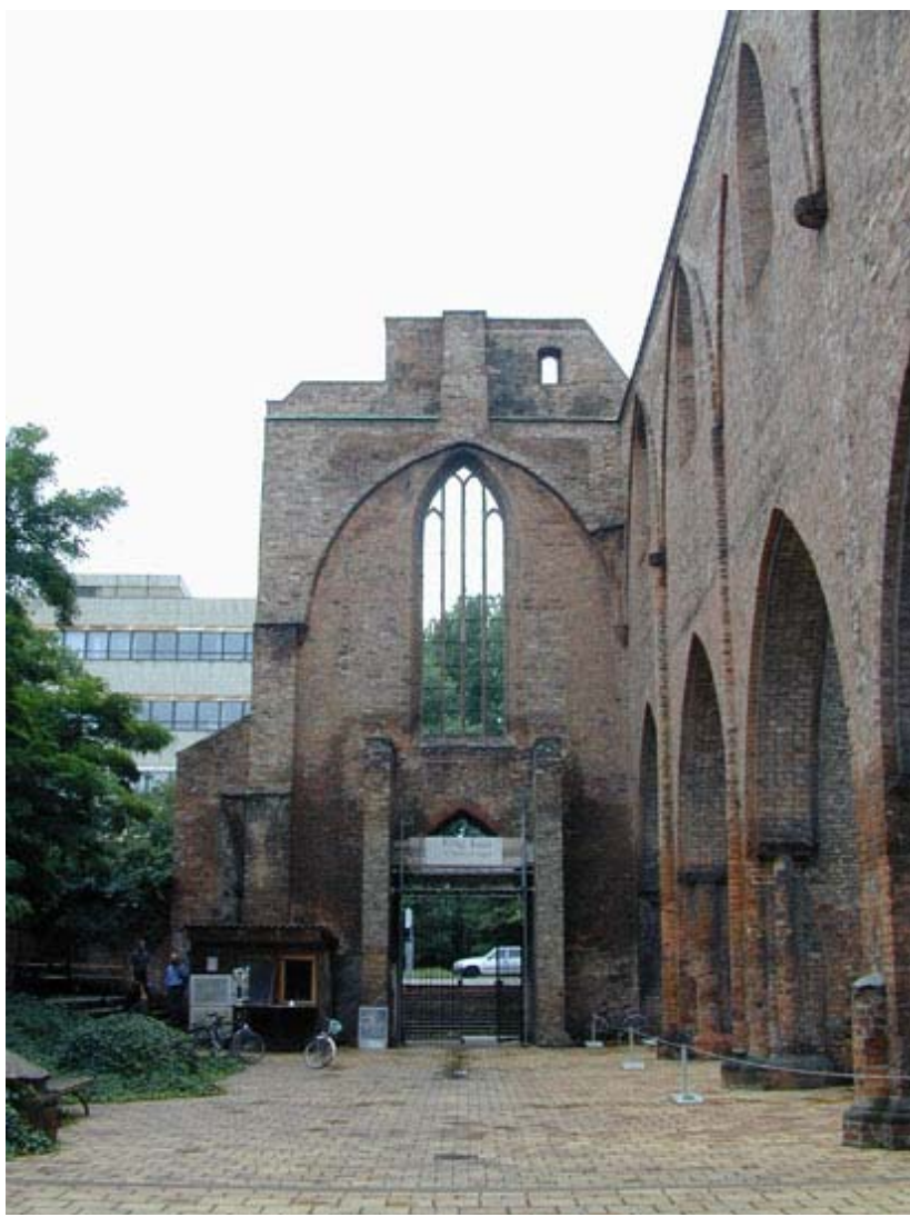
The Kloster ruine, a Franciscan Monastery, was built in the 12th century and heavily destroyed during the World War II. The right side aisle of the basilica and the roof are now missing.
