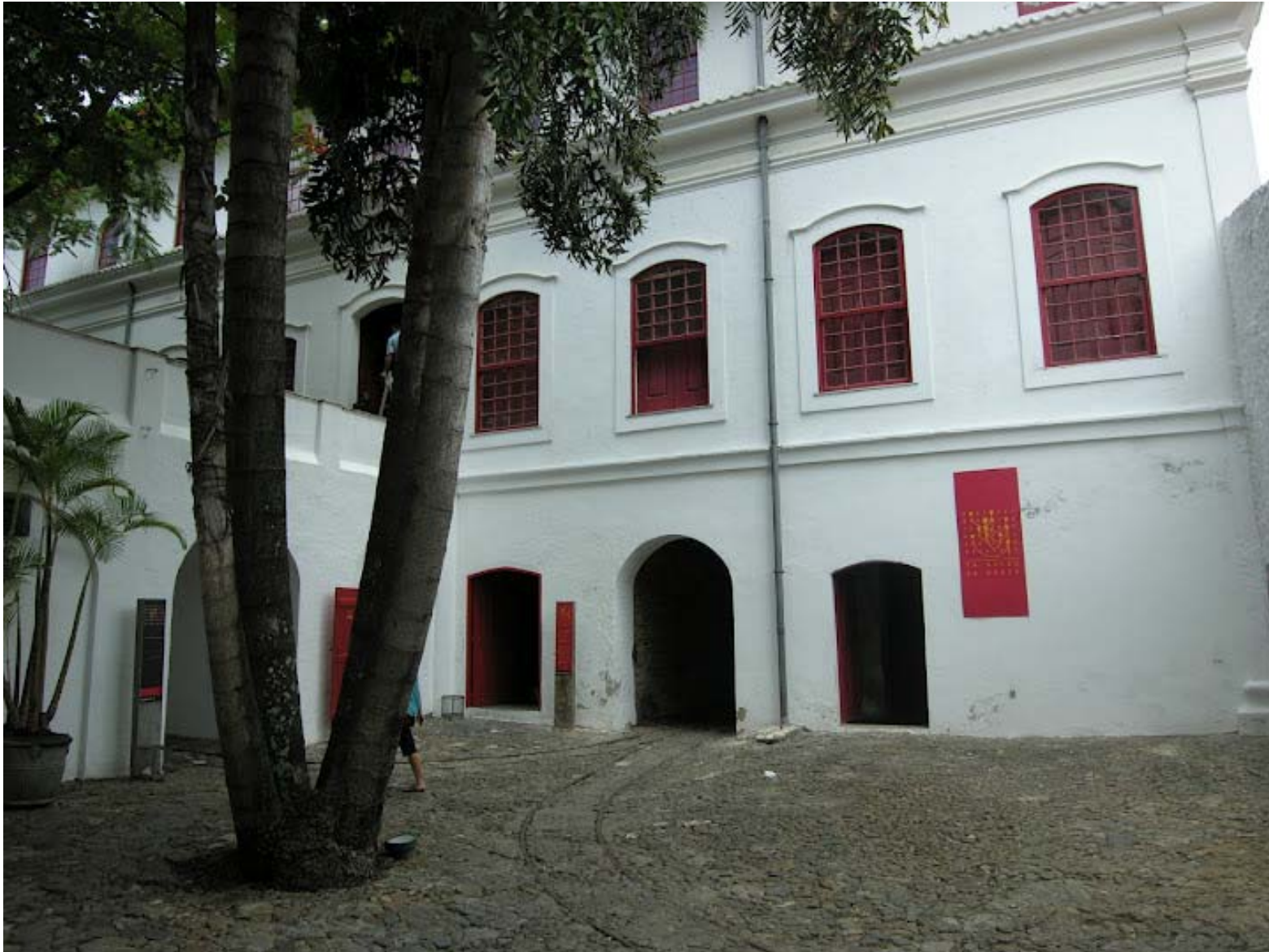
Site view of old sugar factory building.
