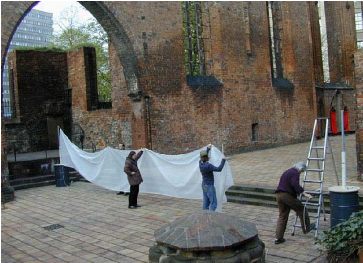
I installed four translucent textiles responding to the original spatial zones. The screens semi-obstruct one's view toward the apse or the exit gate.
